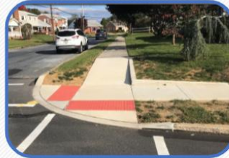
Module 3: HOP - ADA Curb Ramp Design
