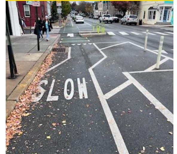
Walnut Street Separated Bike Lane
