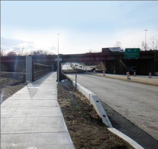
SR 2006, Section 476 - MacDade Boulevard Interchange Delaware County, PA
